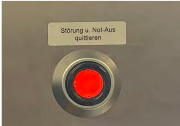
Figure 50: "Acknowledge" illuminated pushbutton
